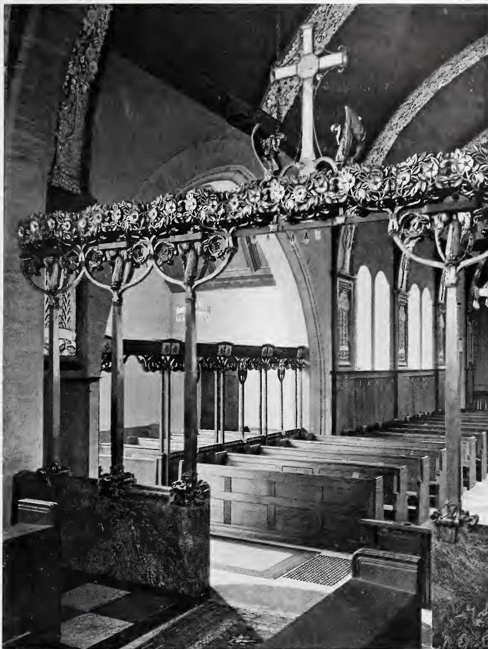
Metal Screen: view from chancel.
